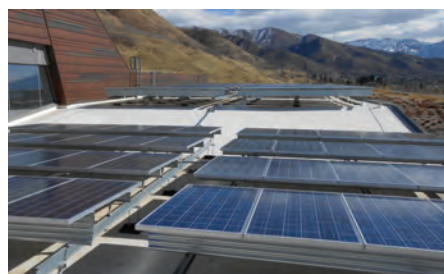
Examples of roof dead loads – HVAC equipment, solar panels and vegetative roofs.
