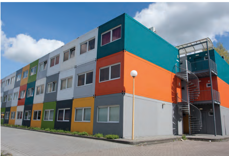
Multi-level structure of intermodal shipping containers.
