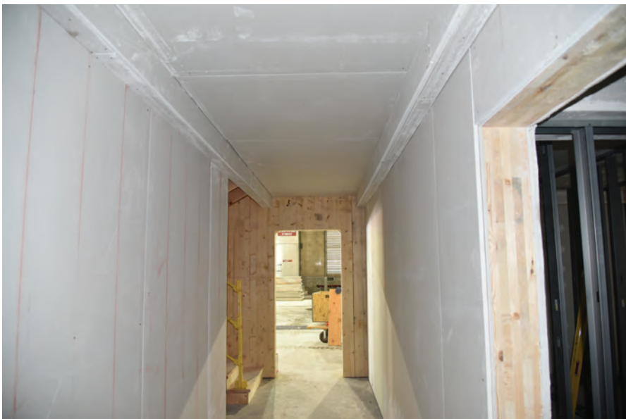
Mass timber and noncombustible protection.
