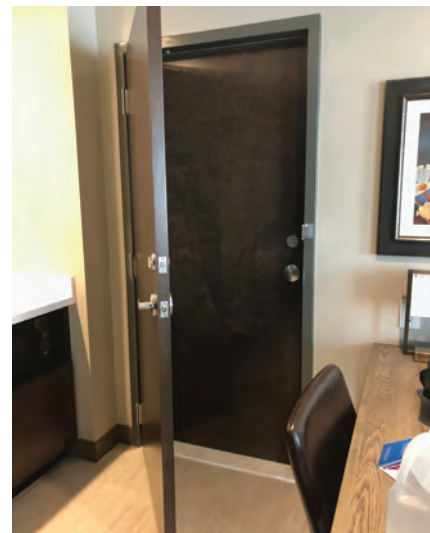
Fire partition with two 20-minute doors.
