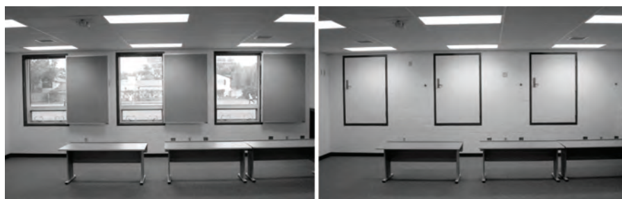
School storm shelter with open and closed shutters.
