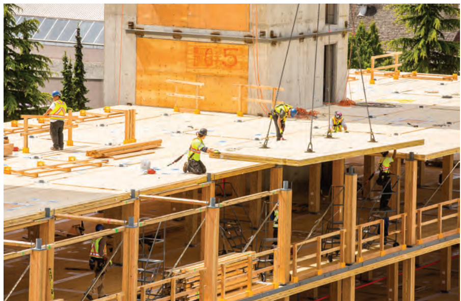
Mass timber construction with glulam and CLT.
