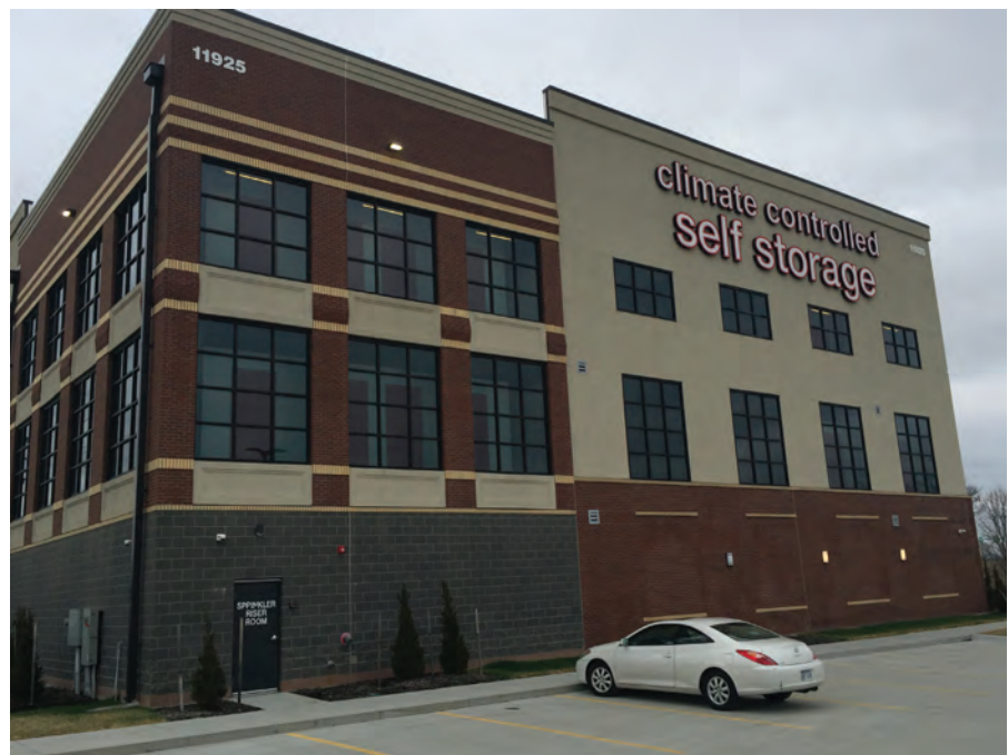
Storage building requiring a fire alarm.
