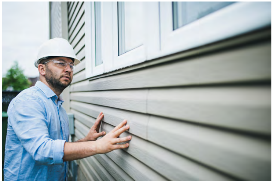
Exterior wall covering example.
