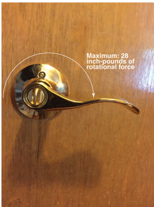
Operational force for door hardware.
