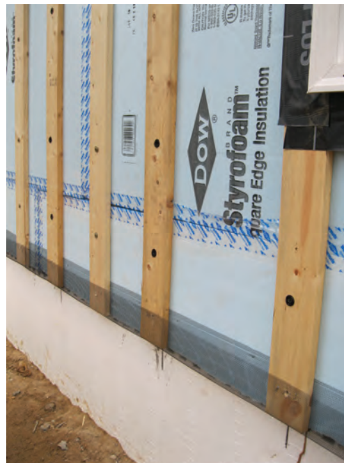
Furring forms a nailable substrate over insulation and beneath vinyl siding.
