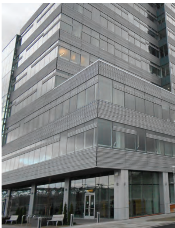
MCM use for cladding of an urban building.
