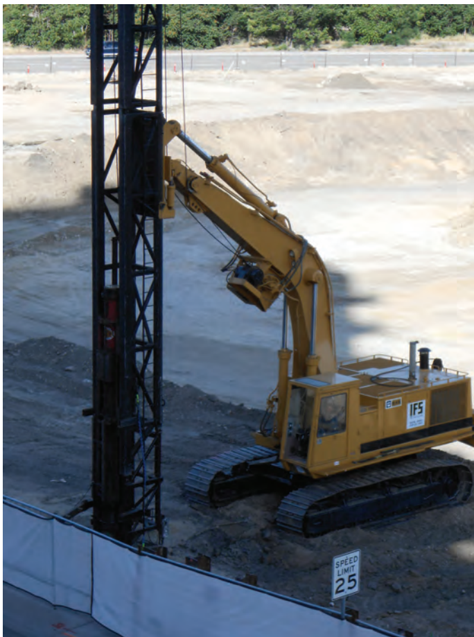
Installation of H-piles.
