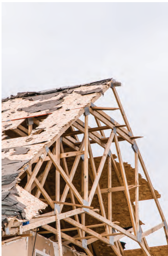
Hurricane winds uplifting roof.
