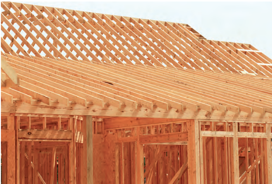
Heel joint connection.
