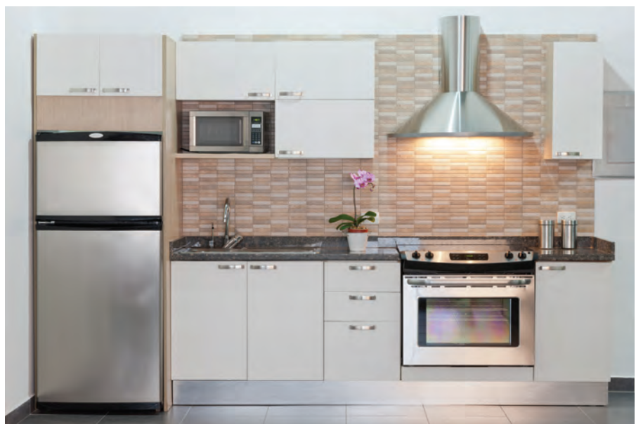
Local exhaust mechanical ventilation for a kitchen substitutes for an openable window.
