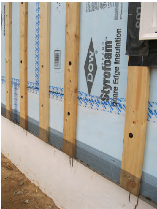
Vinyl siding over foam plastic sheathing.
