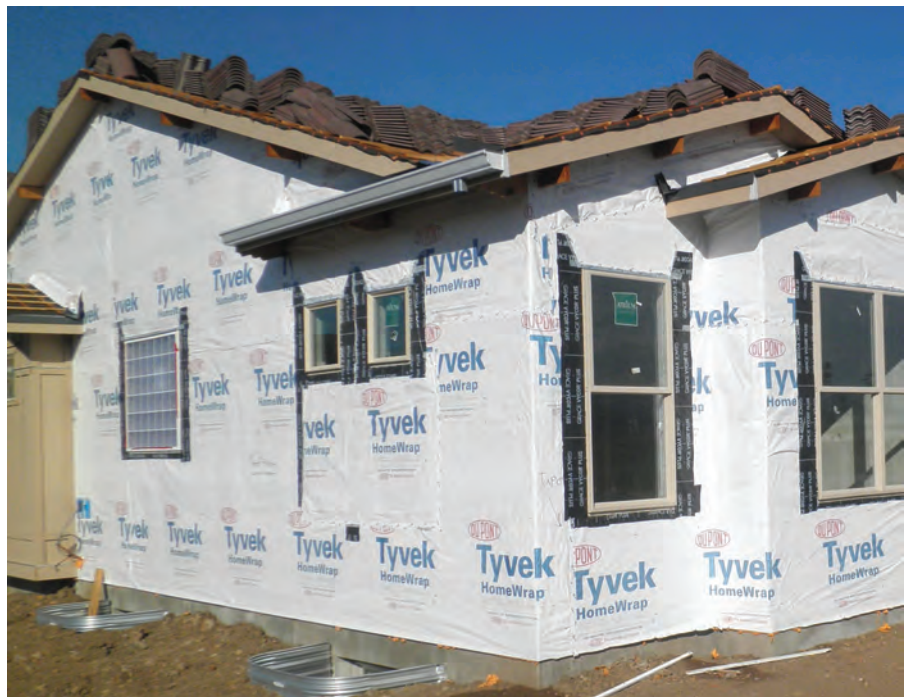
House wrap installed as a continuous water barrier.
