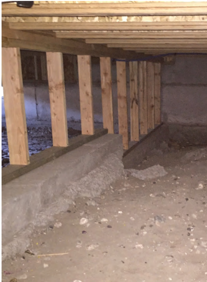
Interior cripple wall.
