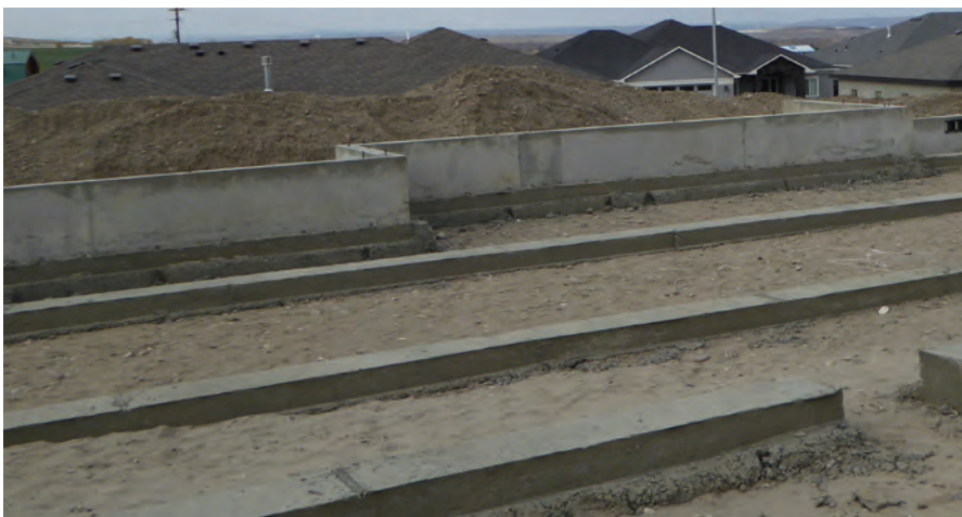
Stem wall and interior footings.
