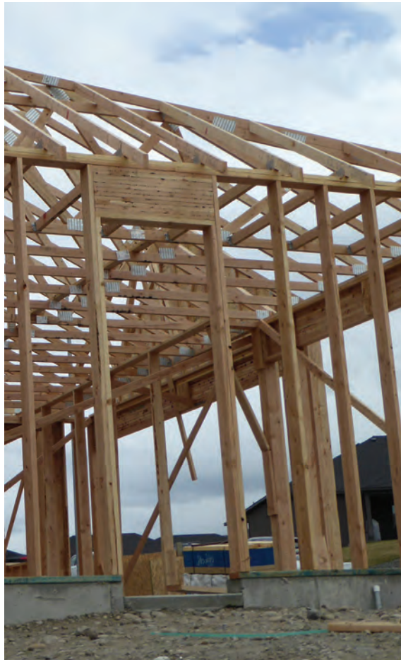
King studs nailed to header.
