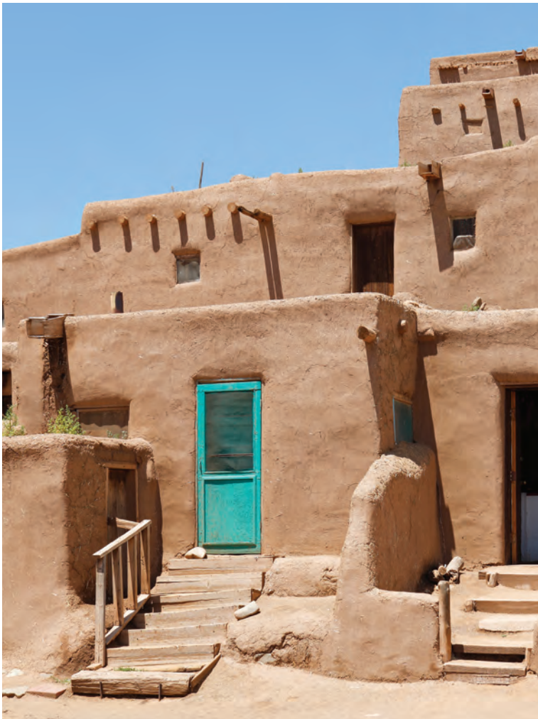
Cob construction with clay exterior finish.
