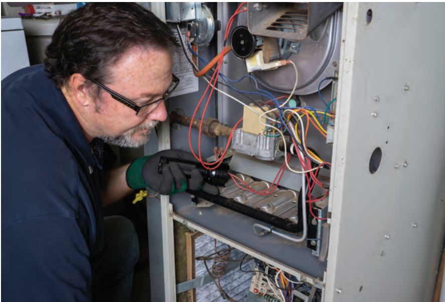
Repair of a fuel-fired furnace.
