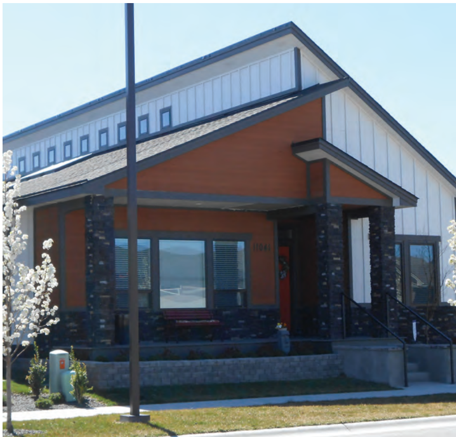
Irregular building shape.
