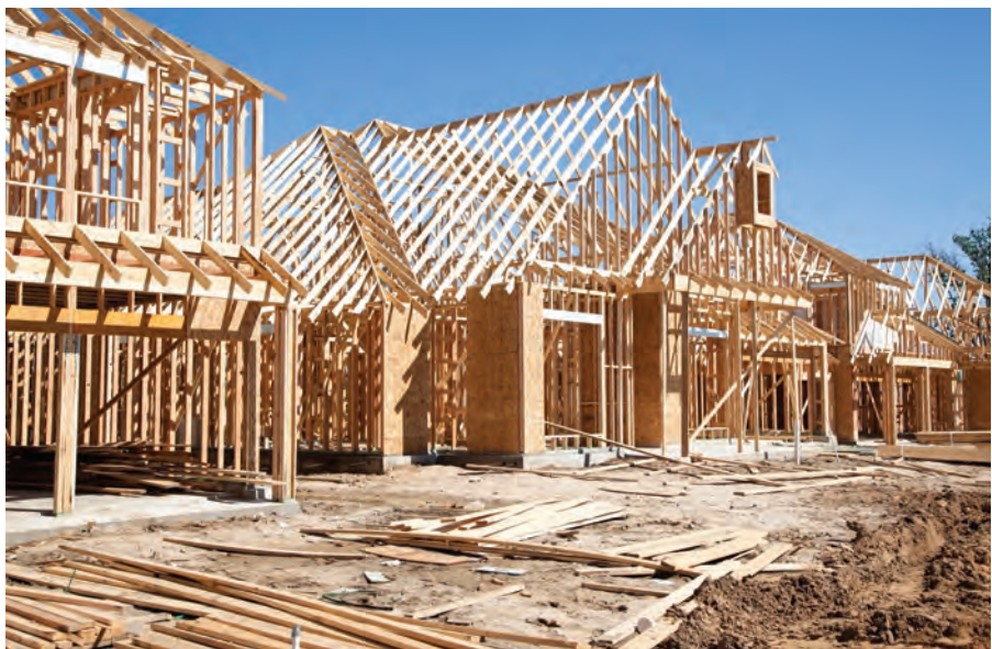
Wood-framed roof line.
