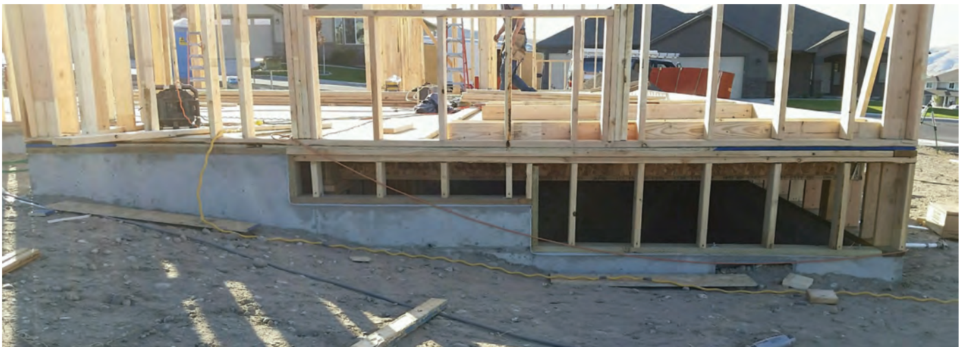
Cripple wall along exterior of house – unsheathed.
