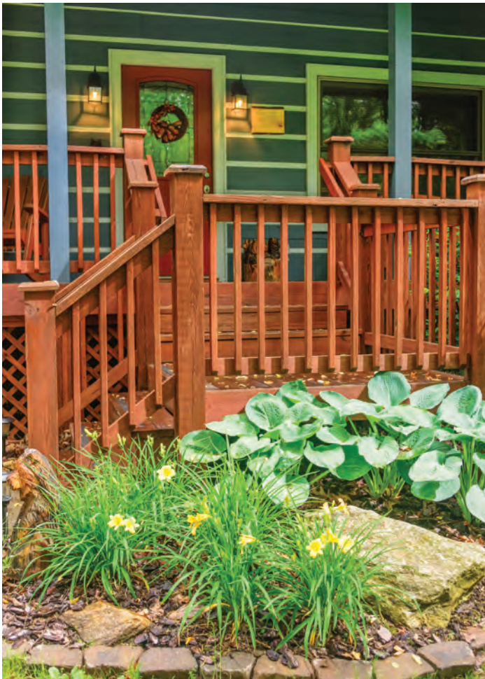
Stairways attached to porches and decks must meet the requirements of Section R311.7.
