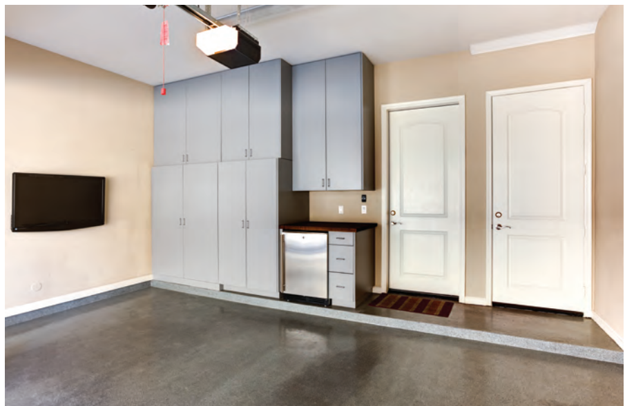
Door from garage to house must be self-closing and self-latching.
