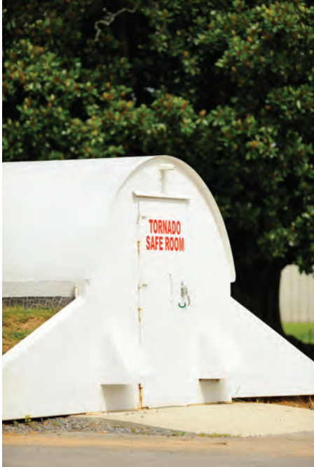
Exterior of storm shelter.
