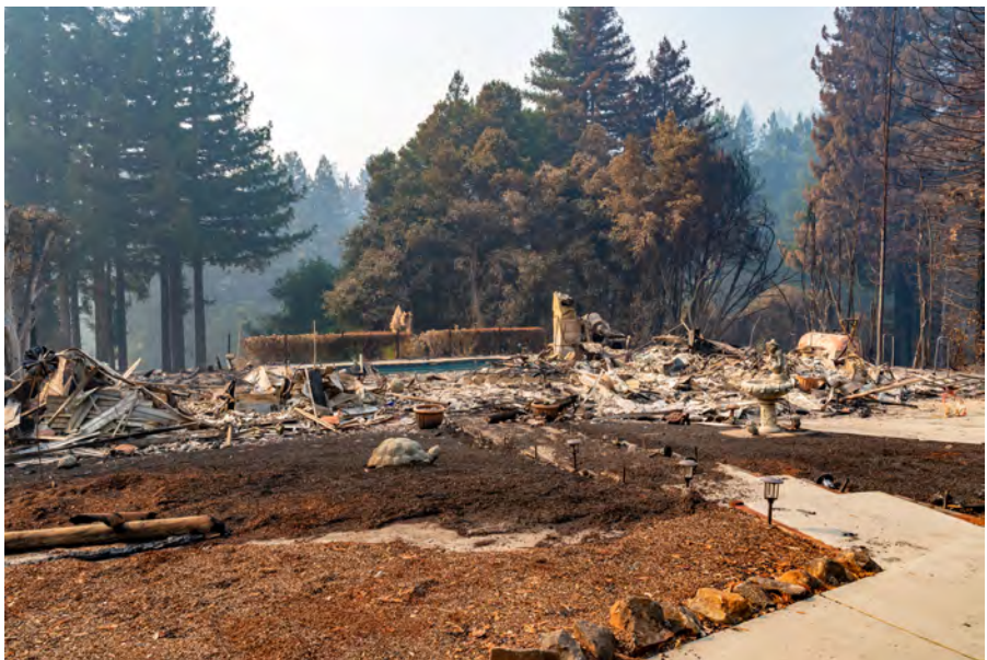
Fire damage from an unprotected structure in the WUI.
