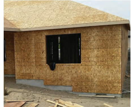
Cripple wall along exterior of house – sheathed.
