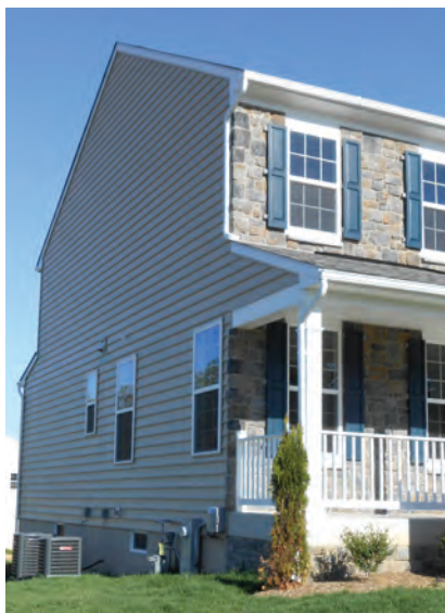
Veneer above first story on one side of the building.
