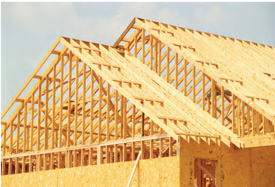
Rafters bearing on exterior side wall.
