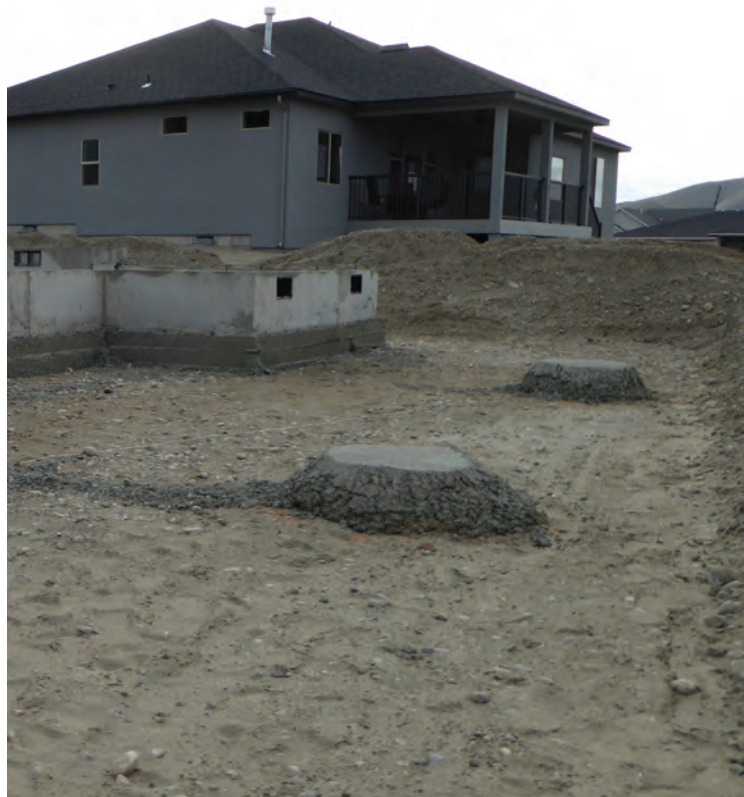
Footings for buried pressure-treated deck posts.
