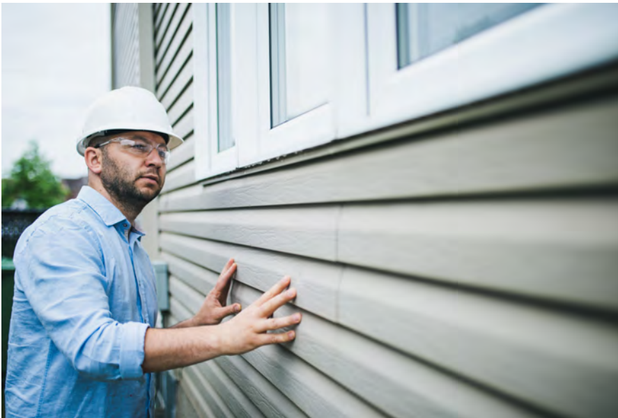
Exterior wall covering.
