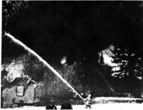
practice burn of existing structures, June 2006
