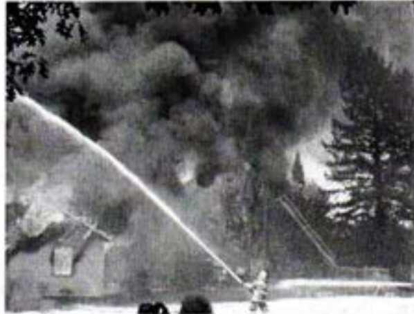
practice burn of existing structures, June 2006
