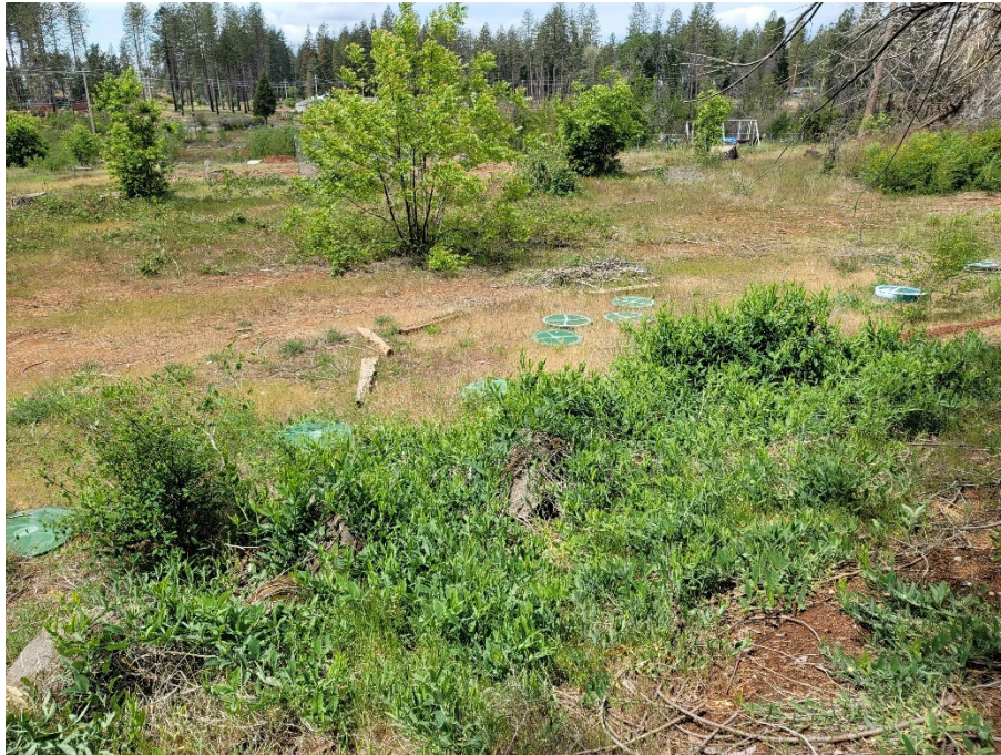
Photograph 9, view facing west: Septic field at 1633 Cypress Lane, APN 050-140-155, north of Cypress Lane.
