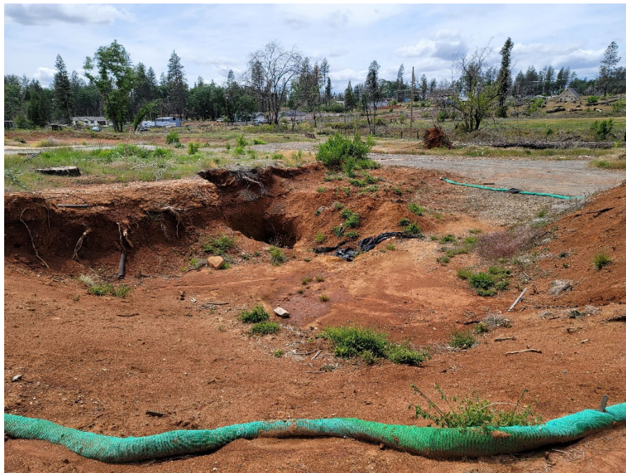
Photograph 16, view facing southwest: 1620 Cypress Lane, APN 050-140-162, UST investigation excavation pit.
