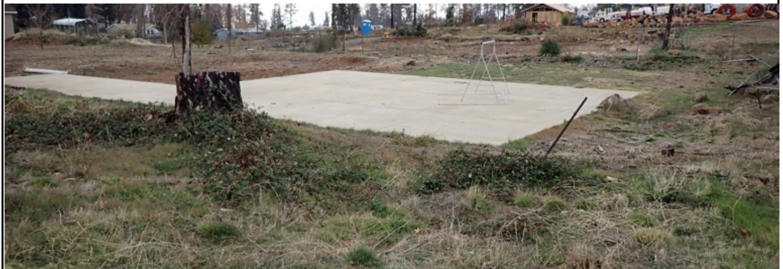
Image 6. Concrete pad observed on the subject property.
