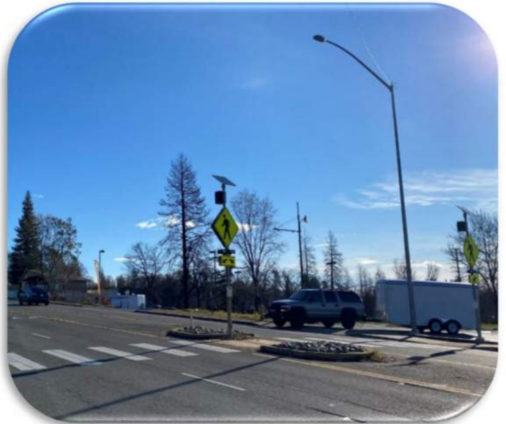
Raised Mid-block Pedestrian Island outside of Paradise Town Hall was removed in 2021
