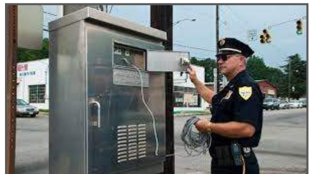
Exhibit 8. Temporary modifications by personnel may increase capacity and flow toward the evacuation endpoints.
