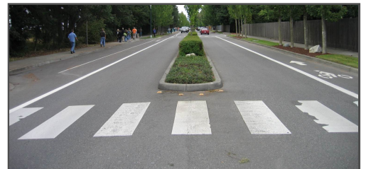
Raised landscaped median. Source: Designing for Pedestrian Safety
