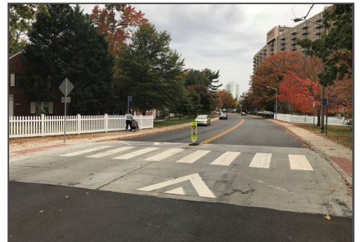
In-street crossing sign at a raised crosswalk in Alexandria, Virginia. Federal Highway Administration.
