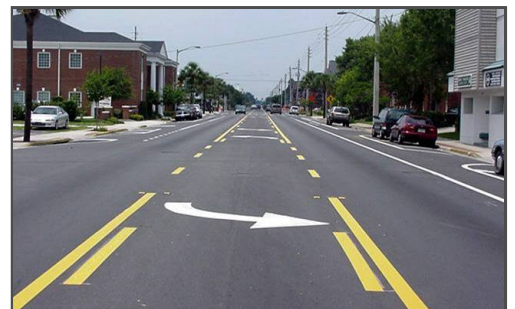
"After" picture from a typical four-lane to three-lane conversion.
