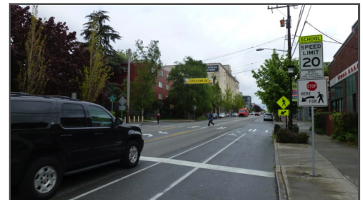
The advance stop bar is supplemented with the “Stop Here For Pedestrians” signs. Source: Toole Design Group.
