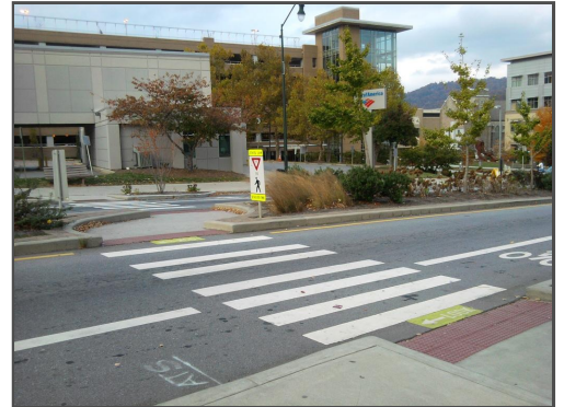
Center crossing islands allow pedestrians to deal with only one direction of traffic at a time, and can be constructed so that crossing pedestrians are forced to the right to view oncoming traffic as they are halfway through the crossing. Source: pedbikeimages.org - Lyubov Zuyeva (2011)
