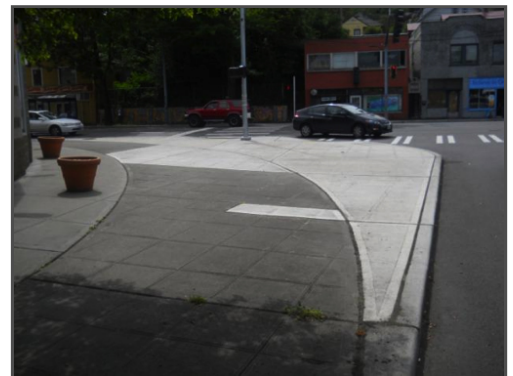
This modified curb radius reduces the speed of turning vehicles and shortens the pedestrian crossing. Photo by Michael Hintze
