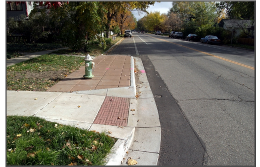
Curb extension in a residential setting. pedbikeimages.org - Dan Burden
