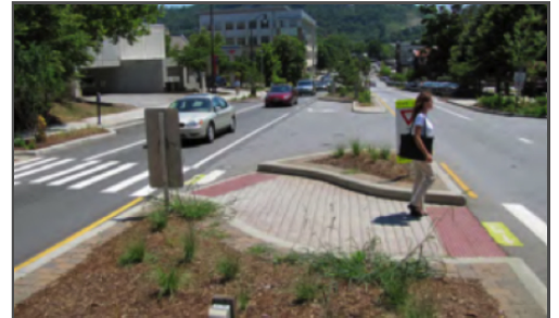
Example of a well-designed right-turn slip lane with a refuge island that forces pedestrians to face on-coming traffic, and marked crosswalks. Source: Living Streets (Dan Burden)
