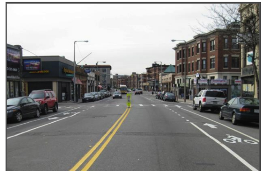
Lane diet on Harvard Ave in Boston, Massachusetts Source: Bill Schultheiss, Toole Design Group
