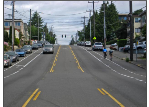
Lane diet (center lane narrowed) creates space to install bike lanes which also provides additional buffer for pedestrians on sidewalks. Seattle, Washington Source: Gina Coffman, Toole Design Group
