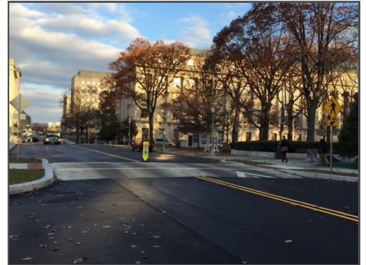
This midblock raised pedestrian crossing features curb extensions and an in-street pedestrian crossing sign. Pennsylvania Department of Transportation.
