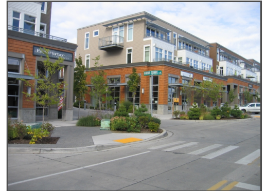
This curb extension at an intersection shortens the crossing distance for pedestrians and creates space for landscaping. pedbikeimages.org - Carl Sundstrom
