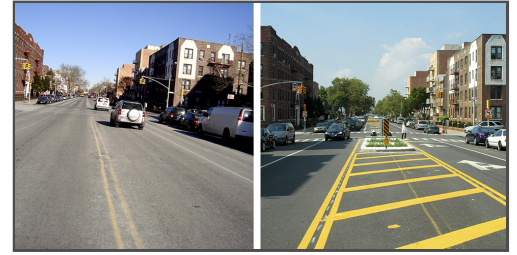
Side-by-side before and after pictures of a road diet with a pedestrian refuge island. pedbikeimages.org - New York City DOT.
