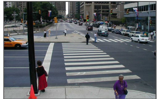
Crossing islands can be located at intersections or midblock crossings to help protect crossing pedestrians from motor vehicles. They allow pedestrians to avoid conflicts with traffic at street level. Source: Designing for Pedestrian Safety
