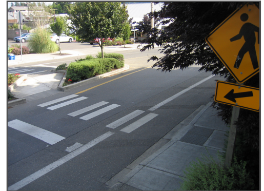
A marked crosswalk with a warning sign and pedestrian refuge island. pedbikeimages.org - Carl Sundstrom
