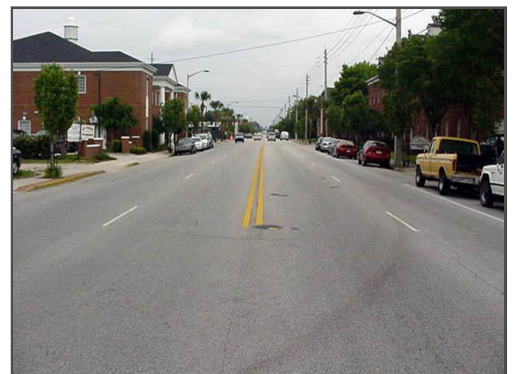
"Before" picture from a typical four-lane to three-lane conversion. Federal Highway Administration.
