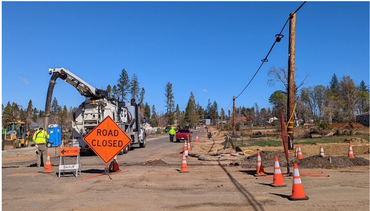
Figure 11 Utility Undergrounding on Almond Road
