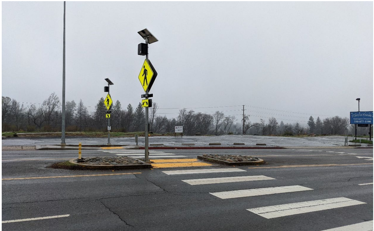
Figure 7 Skyway Raised Median Prior to Recent Removal
