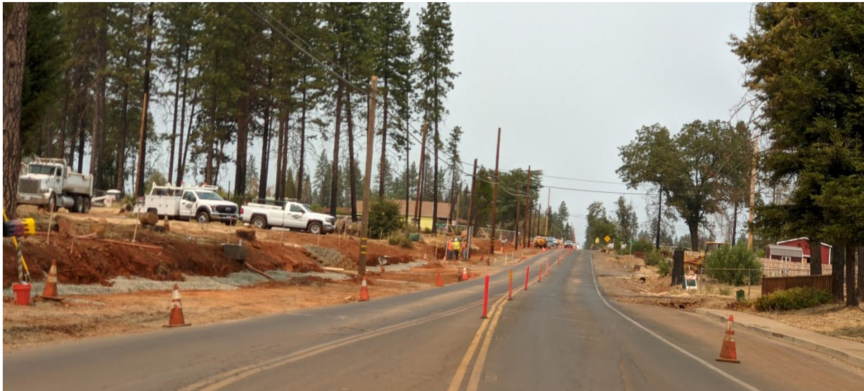
Figure 5 Recent Construction Activity on Pentz Road
