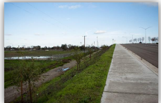
Figure 3 - Capital improvement projects such as roadways must include post-construction design measures and be appropriately sized.
